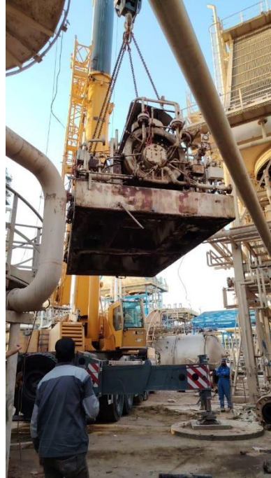
(Gas Compressor Installation – Executed by Our Engineering Team)
